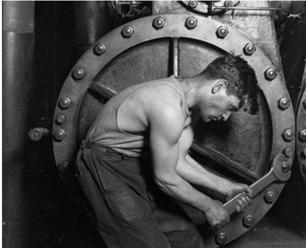
Powerhouse mechanic working on a steam pump Lewis Hine 1920
